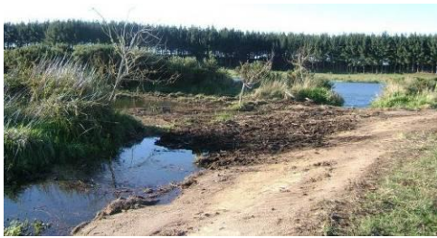
Photo 8. Sill at E2, just completed
