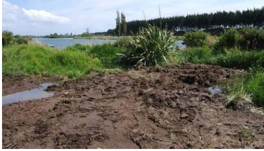
Photo 6. Sill at E1, just completed.
