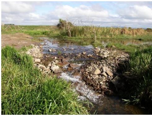
Photo 16. Rock protection of the outfall at E2.
