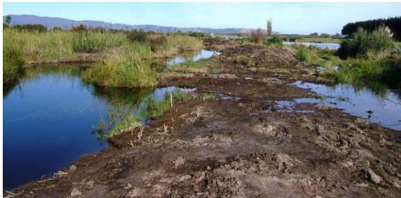
Photo 10. Sill at E3, just completed, high tide moving across.
