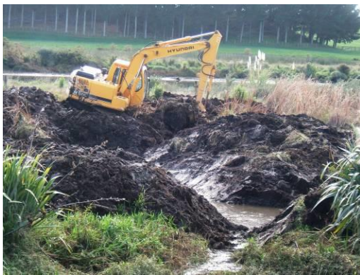
Photo 3. Creating the first new pond.
