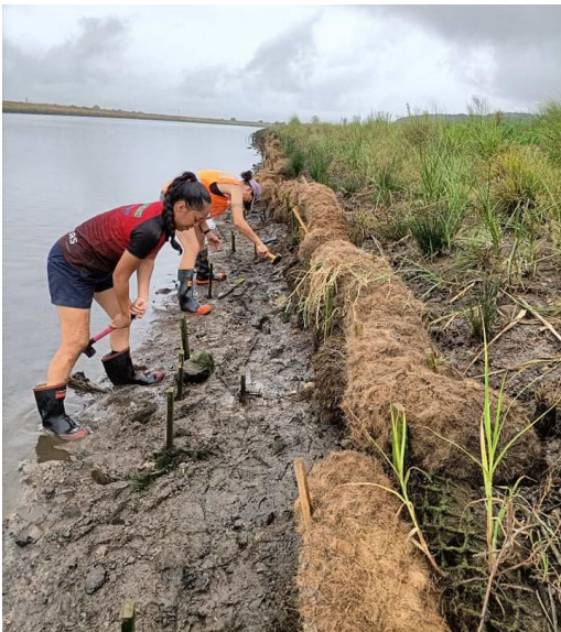
The team undertaking some hard mahi to repair the coir logs at Ford Island in an attempt to prevent erosion (Left – Raven and Awhina; Right – Peter).
