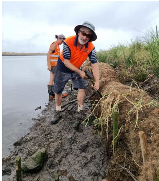
The team undertaking some hard mahi to repair the coir logs at Ford Island in an attempt to prevent erosion (Left – Raven and Awhina; Right – Peter).
